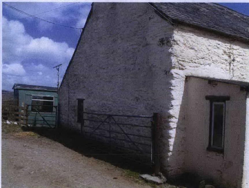
Photograph No.2 WEST ELEVATION
