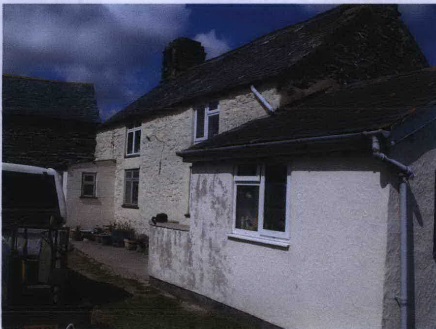
Photograph No.1 SOUTH ELEVATION
